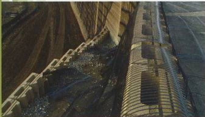
Tensar® Geogrids are used to reinforce the Mesa® Retaining Wall Systems.
